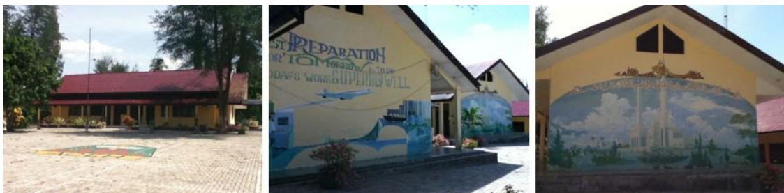
Figure 2. Banda Aceh School. Left: Banda Aceh school's assembly field, used for weekly flag ceremonies. Middle: Building wall facing assembly field. Right: Wall on building opposite to middle picture.
